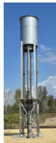
Over the next couple of months, residents may notice a new flame burning at the Regional Water Reclamation Facility. This flame will come from a flare, which is part of our new gas system being installed as part of the facility's expansion.
