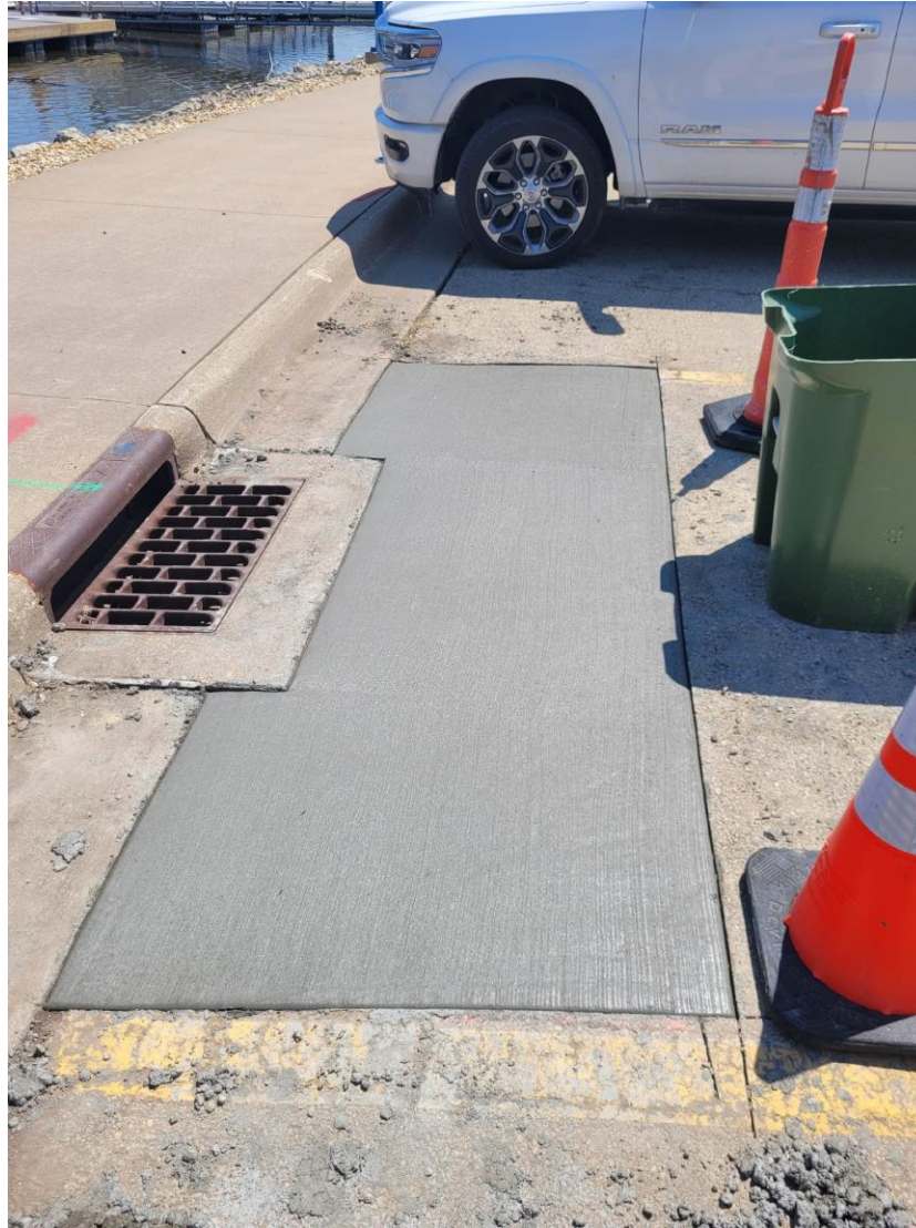
Catch Basin Repairs
