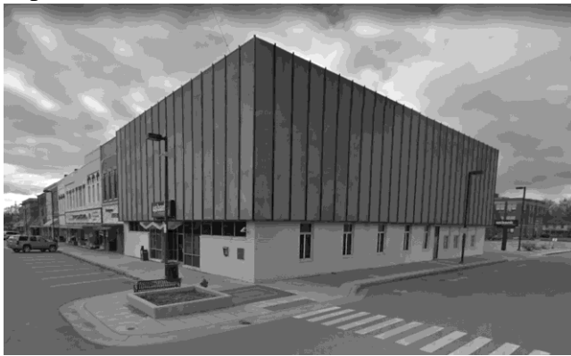
Example of Metal Siding Covering Upper Façade
