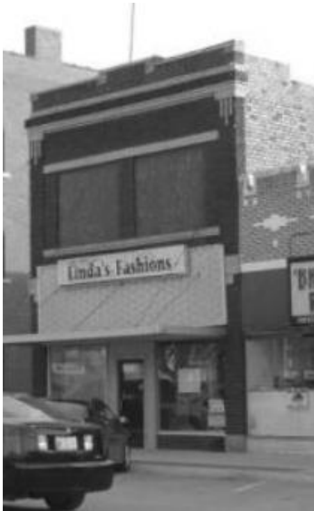
Example of Windows Infilled and Sign Frieze Covered
