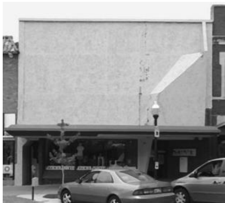
Example of Upper Façade Windows Removed and Covered
